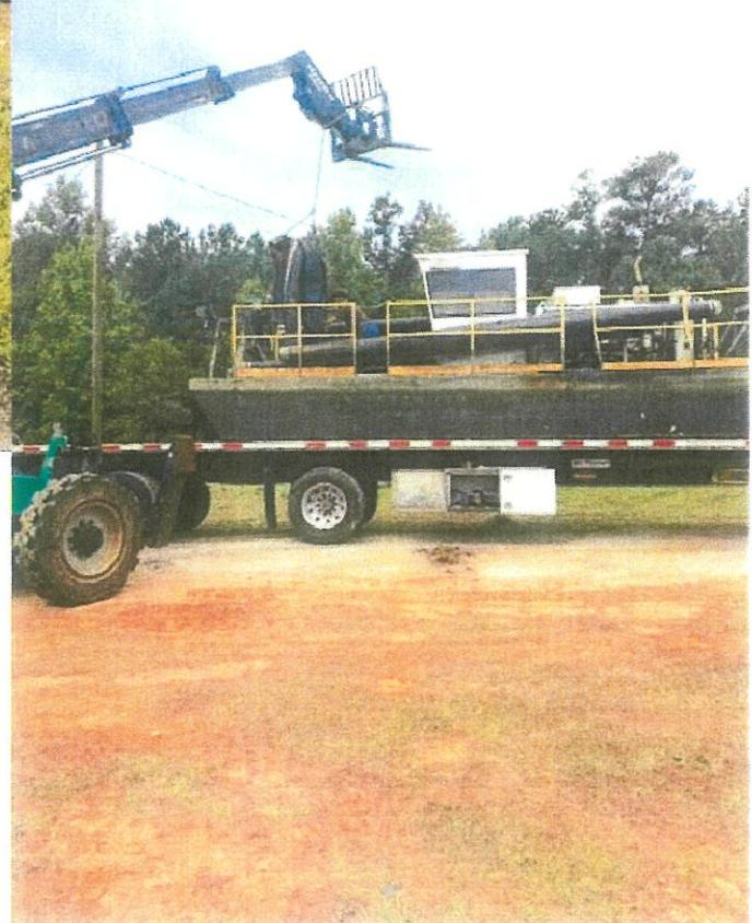
The belt press was also loaded onto a separate trailer and prepped for transport. Power had been disconnected the week prior when the mixing tank was removed.
