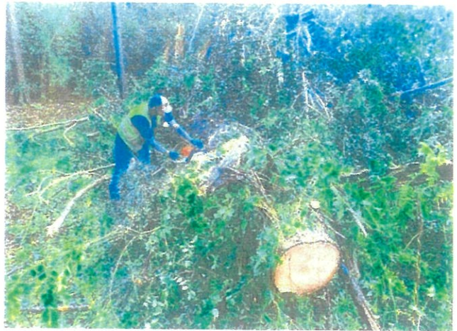
Street department working on clearing the tree on Spring Street.
