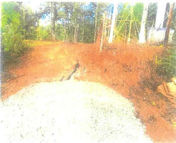
Road repaired at Dixie water tower after heavy rain
