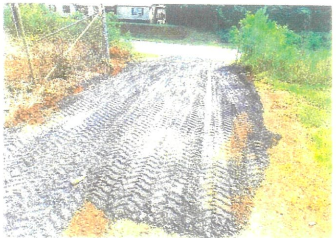
Road at water tower after repair
