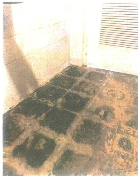
Bathroom Floor – Removing Adhesive
